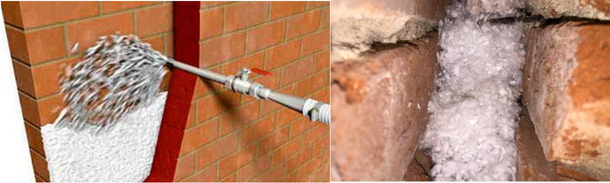
Figure 10. Cavity wall injection (left), view in the insulated cavity wall (right).
