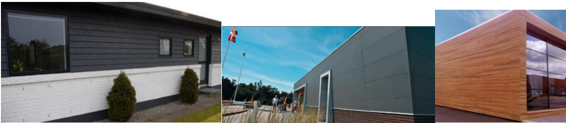
Figure 52. Three finish materials for light external wall: timber (left), fiber boards (middle), cedar wood (right).
