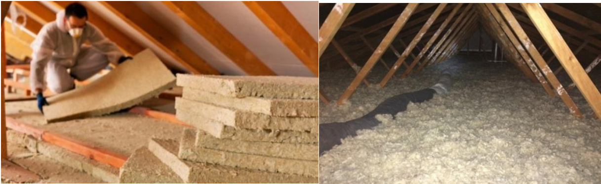
Figure 26. Mineral wool mats (left) and granulate mineral wool blown insulation (right).
