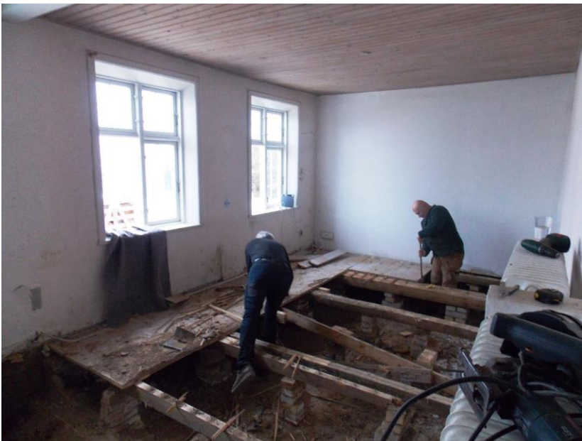
Figure 33. Demolition of not insulated floor above unheated crawl space.
