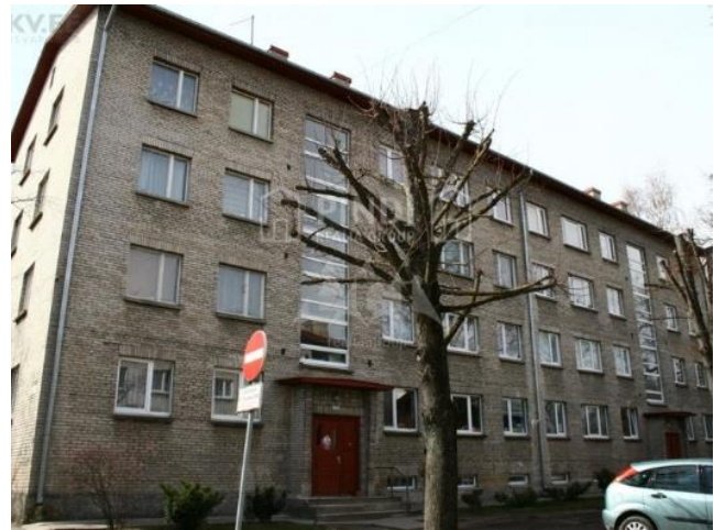
Figure 22 Building in need of refurbishment 3-7 Tiigi street, Tartu
