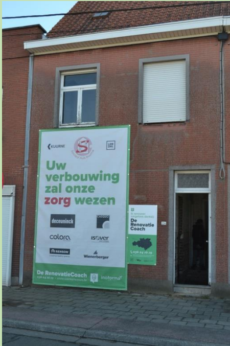
Figure 11 The model renovation in Kuurne
