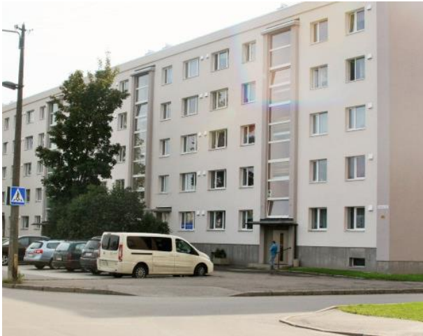
Figure 21 Renovated building 47 Ann street, Tartu
