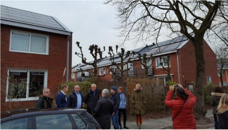
Figure 23: Frisian social rental renovated houses
