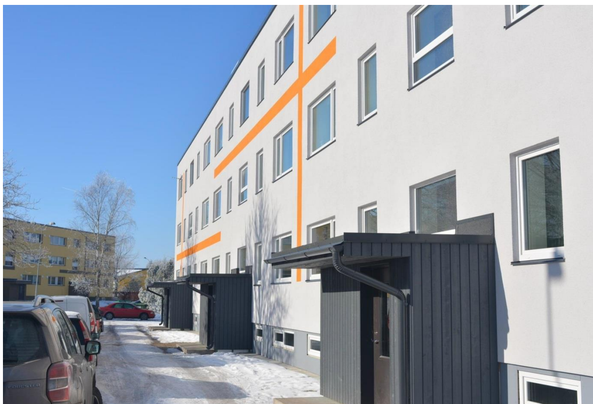
Figure 9 Pilot 2 dwelling Estonia after renovation
