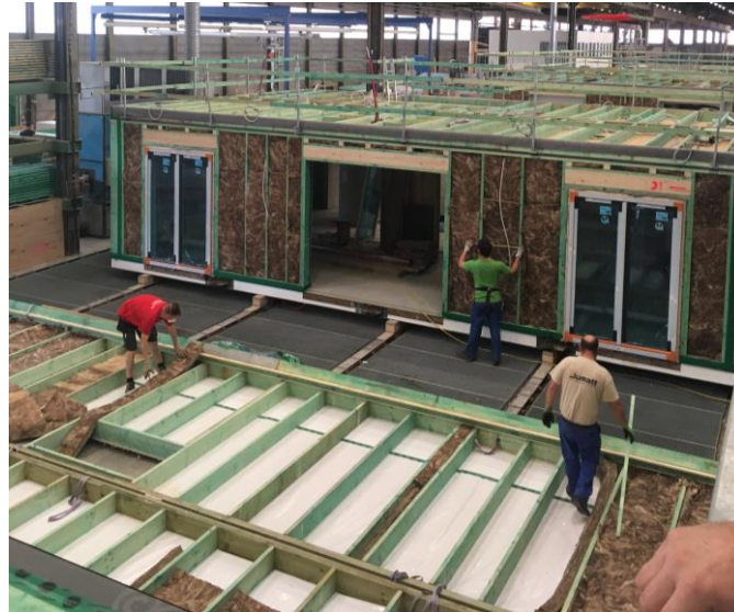
Figure 26: Illustration of timber frame module in production (source: Bostoer)
